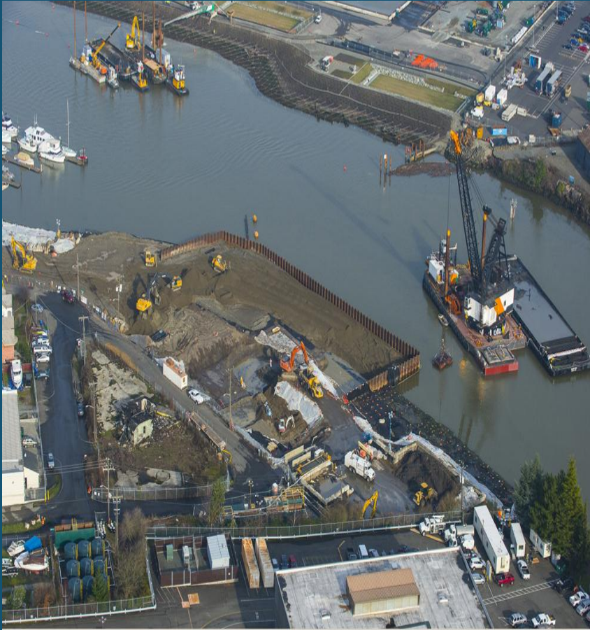
T-117 uplands/sediments cleanup, looking NE to Boeing Plant 2
